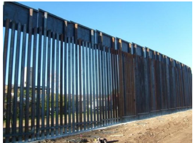
EXHIBIT 1: 18ft tall primary fencing is already used along the US-Mexico border in many urban areas.
